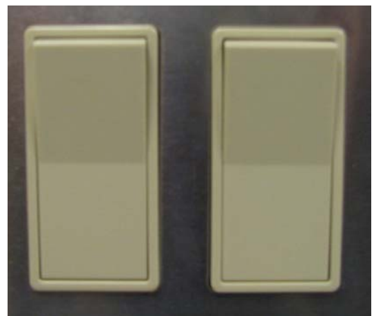
Plate rocker switch- less force and no grip required
